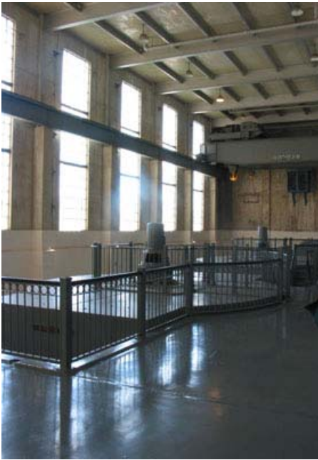
Interior of PK Hydroelectric Powerhouse
