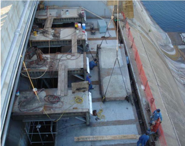
Possum Kingdom Lake gate replacement
