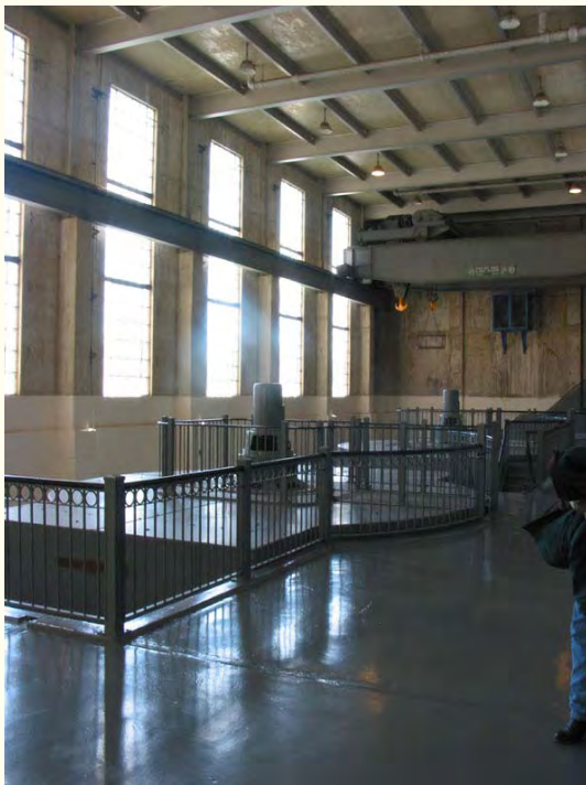
Interior of the PK Hydroelectric Powerhouse
