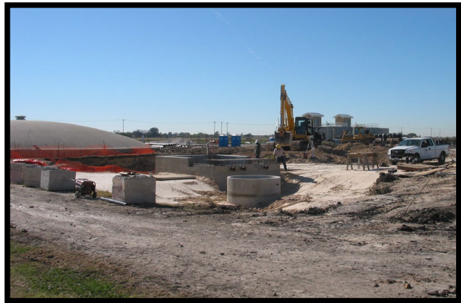
East Williamson County Plant Expansion
