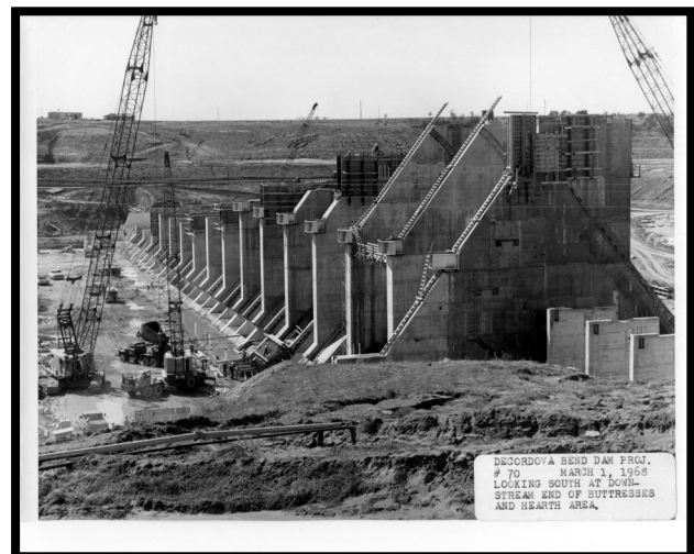
Lake Granbury – Dam Construction
