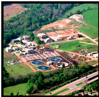
Brushy Creek Regional Wastewater System
