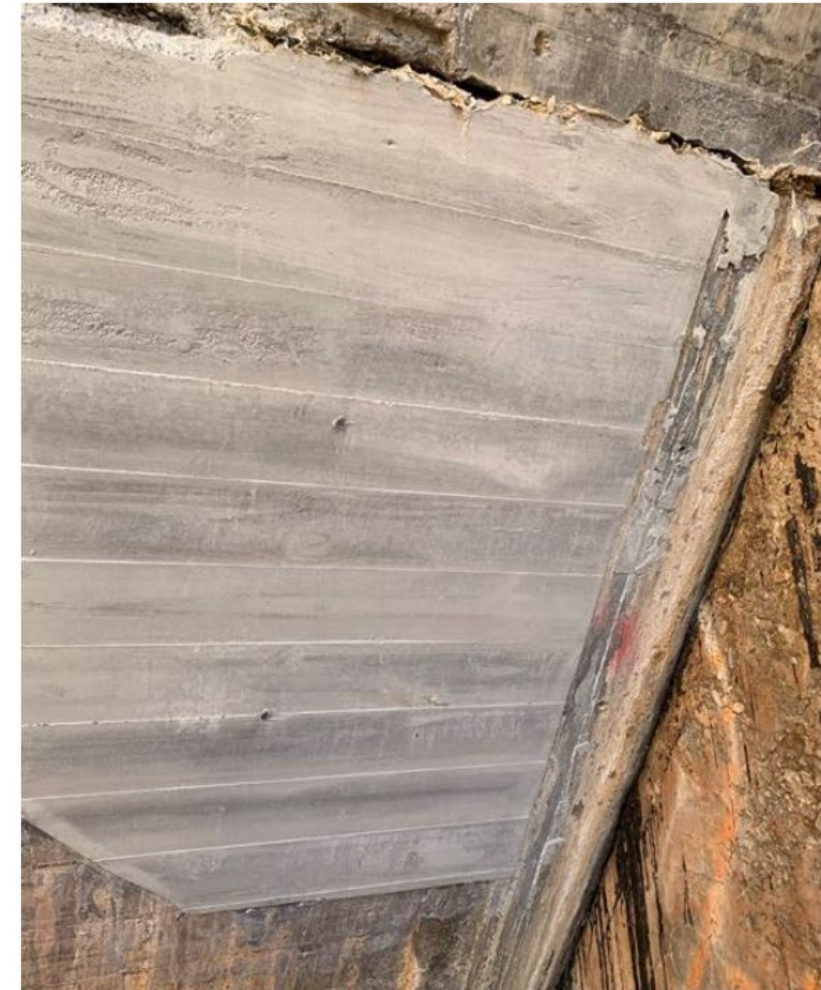
Photo 3-2: Example of Destructive Investigation of Bay 31 Slab 6, March 2022; Concrete Backfilled
